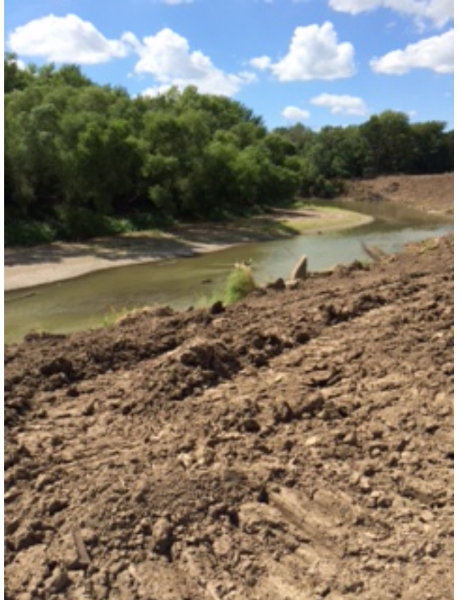
Site 9 – NW View
