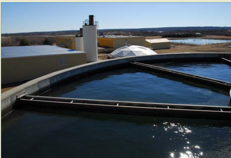
Tri-District Clarifier. Photo courtesy Dennis Schwartz
