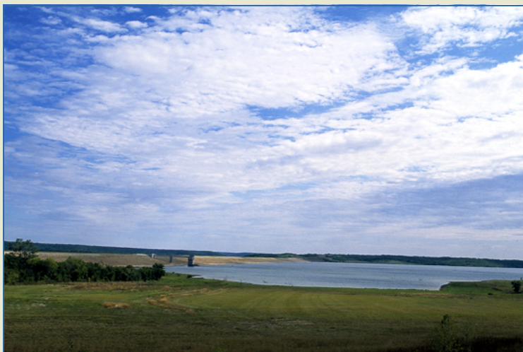
Clinton Dam. Photo courtesy Kansas Geological Survey.
